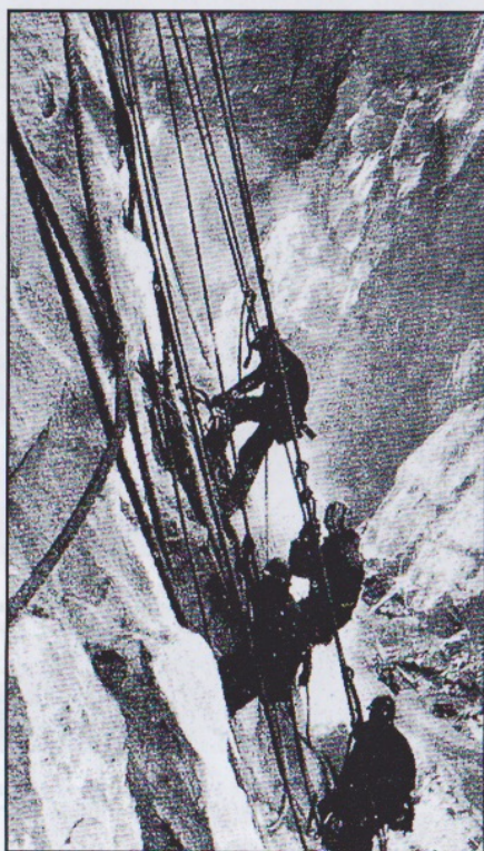
Cuts in the canyon walls for all structures were excavated by high scaling methods
