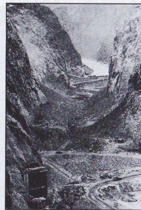
Rock shot down from canyon walls was removed by power shovels and fleets of trucks
