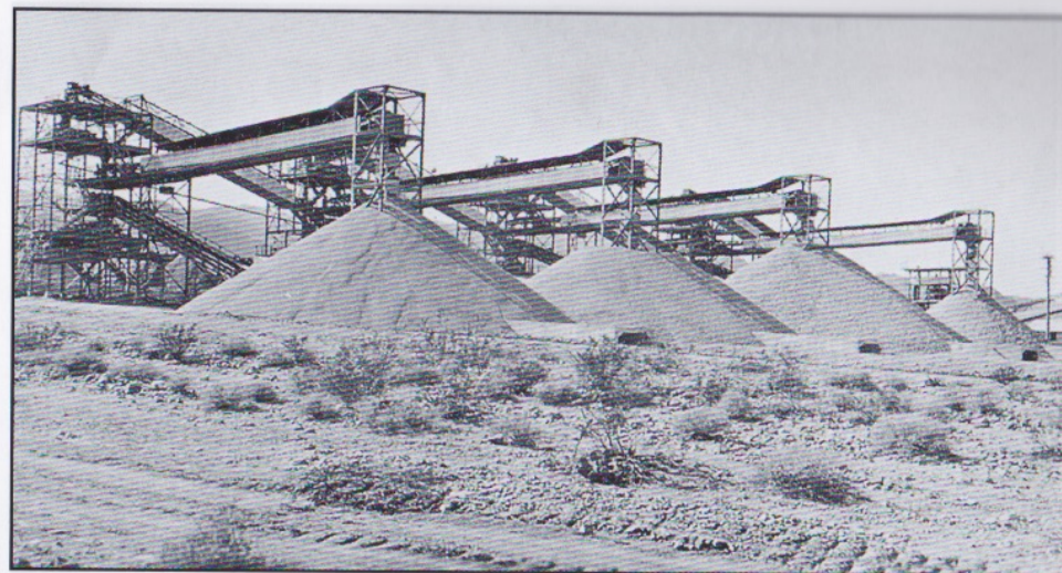
Materials from the pit were separated into different sizes at the screening and washing plant in Hemenway Wash
