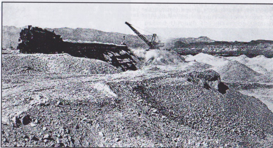
Sand, gravel and cobbles for concrete were secured from a pit ten miles from the damsite
