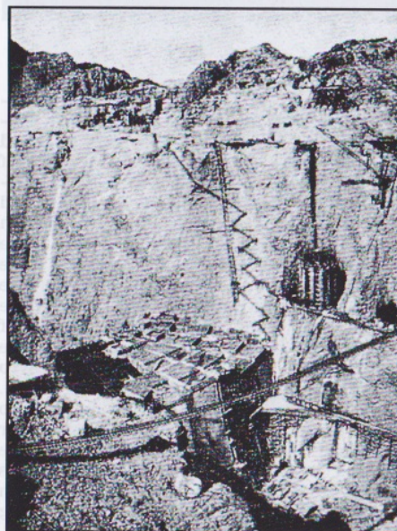
Nine months after the first bucket of concrete was poured, the dam had reached a height of 300 feet
