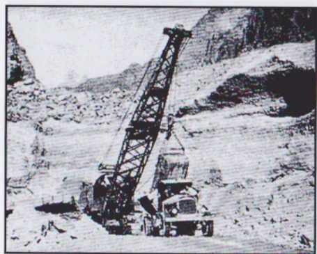
Excavations for the dam and powerhouse proceeded downward below the river bed, toward bedrock
