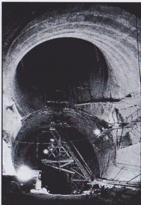
The outlet for each spillway was through a 50-foot diameter inclined shaft which connected with an outer diversion tunnel
