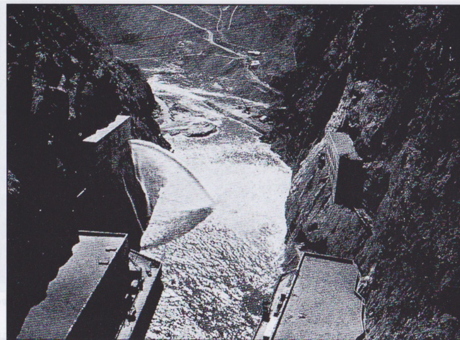
Needle valves of 84-inch diameter located in the valve houses supplement the flow of water downstream from the powerhouse turbines
