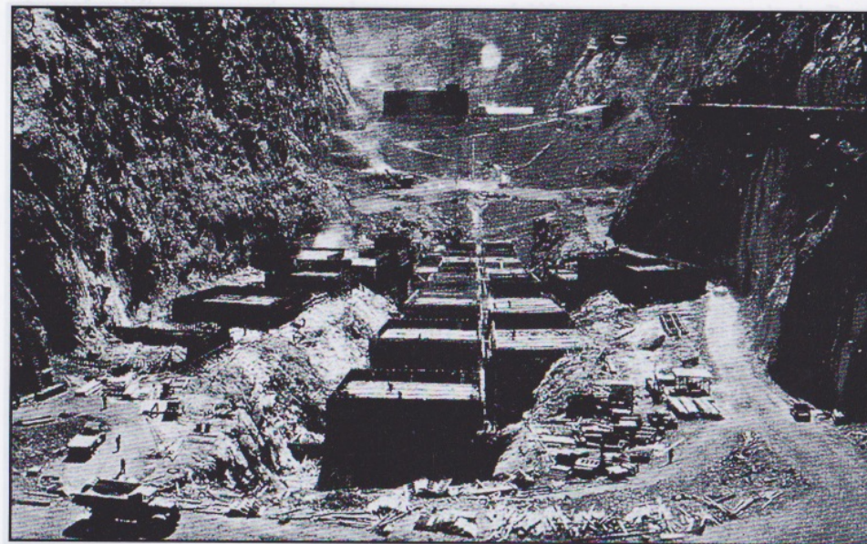
The dam was built as a group of vertical columns closely keyed together
