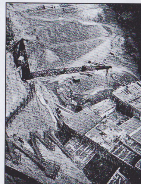
A crane was installed to supplement the cableway operations. This view is from the top of the Nevada abutment and toward the upstream face
