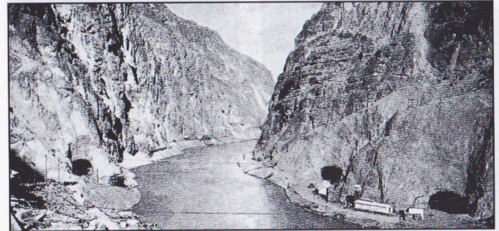
Diversion tunnels were driven through the canyon walls around the damsite. The outlet portals of three tunnels are shown
