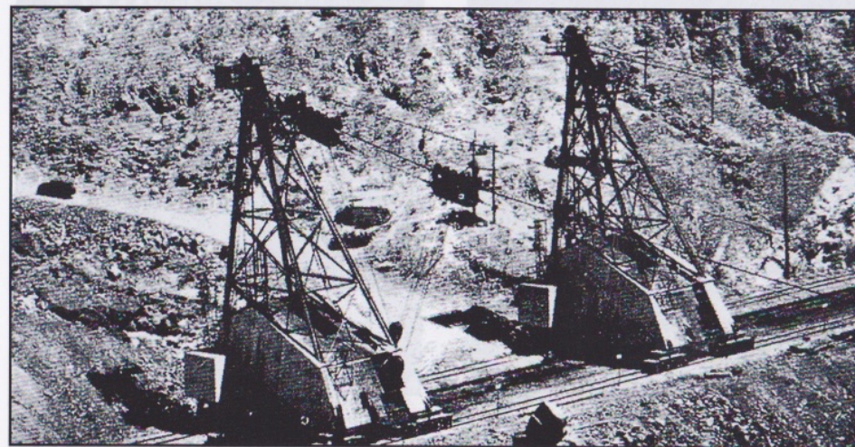
A group of cableways with traveling end towers were installed to transport concrete and other materials from canyon rim to pouring site
