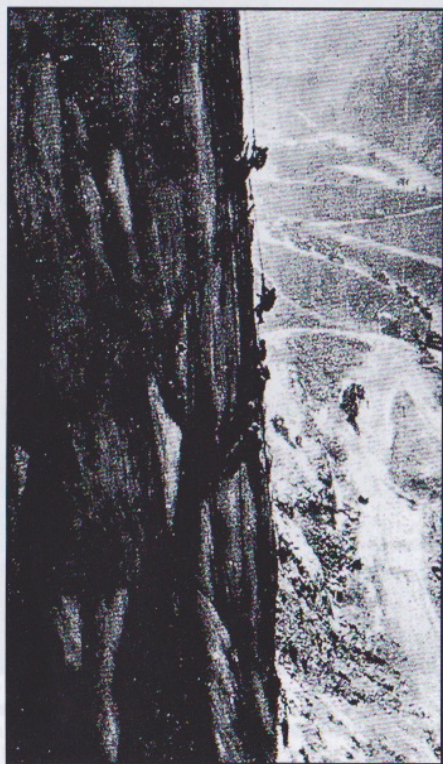
Both canyon walls were stripped of loose rock by the "High Scalers"
