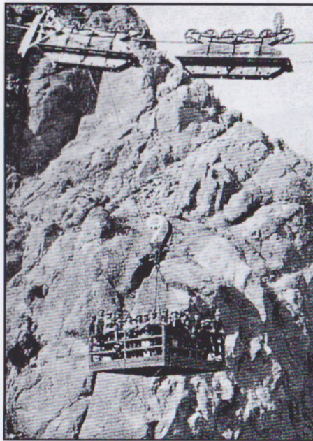
Men and materials traveled by cableway from canyon rim to locations on canyon walls
